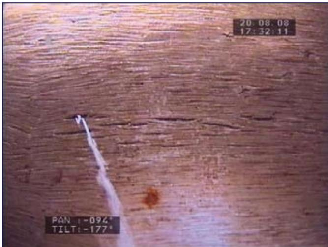
Figure 3. Bubble jet on the inside of the cooling circuit, at the reducer position.
